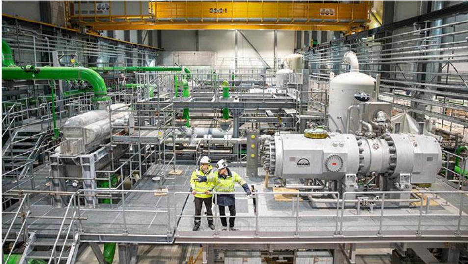
Figure 1. Example image, not exhaustive, just for illustrative purposes of MAN Industrial Heat Pump installed in the modern heat pump hall near the Esbjerg Harbor (Denmark) [4], which houses the world's largest sea-water (Renewable Energy Source according to RED Directive) heat pump, which replace coal-fired heat plant for district heating application. Electricity for the heat pumps is generated by giant offshore wind farms, producing an abundance of clean energy, making the district heating 100% renewable.
