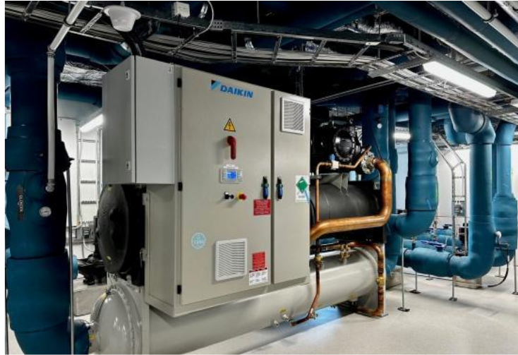
Figure 5. Picture for illustrative purposes (non-exhaustive) from Daikin Applied Europe S.p.A. of High Temperature HP Water to Water EWWH- VZ with nominal heating capacity (depending on the size and features selected) from 400 – 1900 kW, using low GWP Refrigerant, R-1234ze, with Inverter-driven Screw Compressor. It can be suitable for use in several applications of waste heat recovery. With “modular combination”, they can scale from 2 to 10 MW and more of heating capacity with stable and reliable technology [19]
