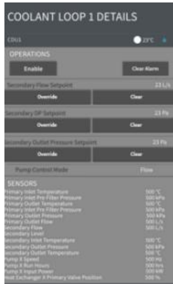
Figure 65 – Colling Distribution Unit Data
